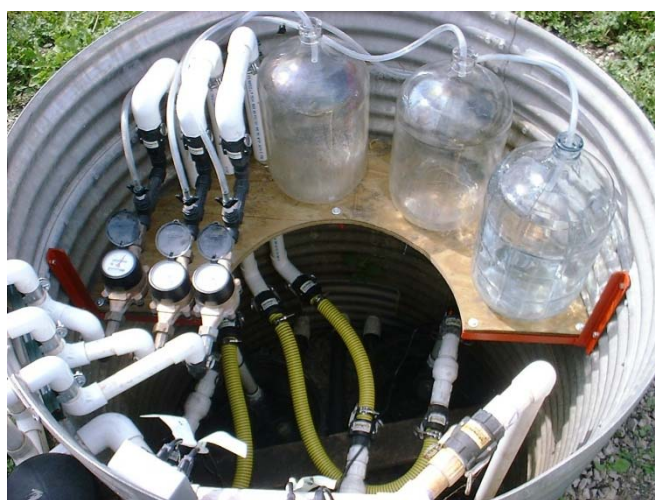
Figure 3. Drainage monitoring sump configuration
